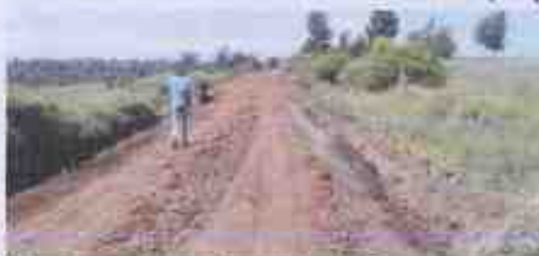
Ongoing road opening in Mukogodo East
