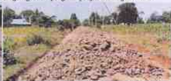
Ndaragwiti-Wangaci & Sipili Pry School Ribs - Ol moran
