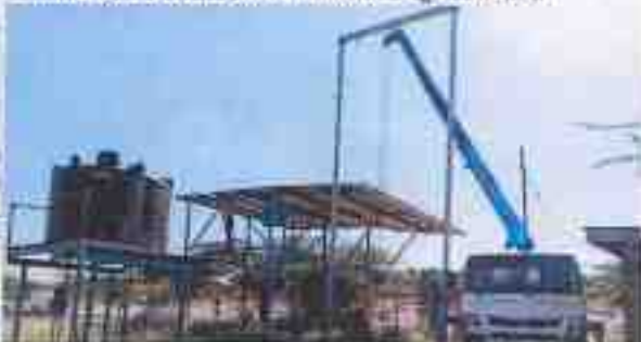
Rehabilitation of Naiperrre 2 borehole, Laikipia
