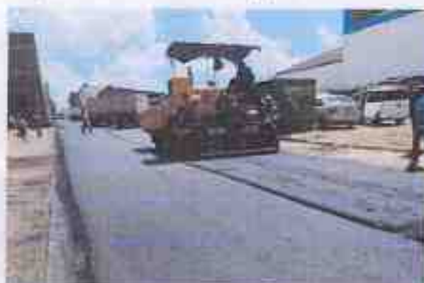
Overlaying of tarmac in Nyahururu town, Igwumiti
