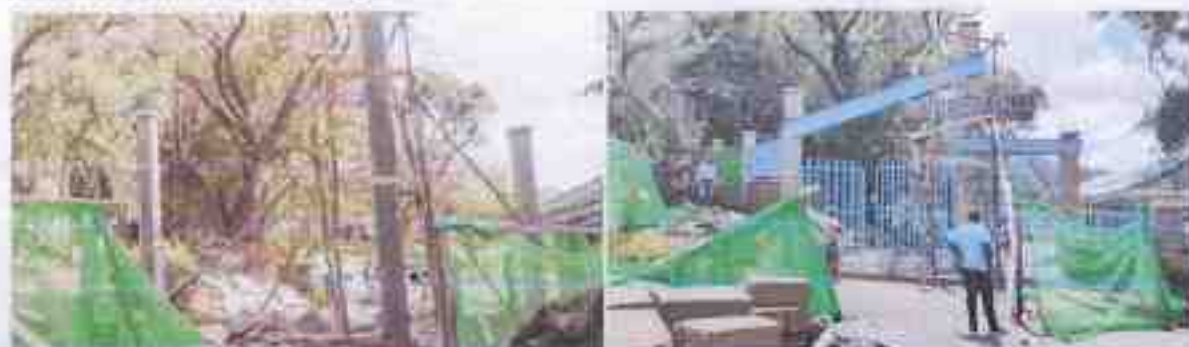
Renovations of Open Air Market, Nyahururu town
