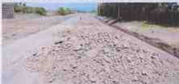
Olpejeta road, grading and gravelling- Tigithi ward
