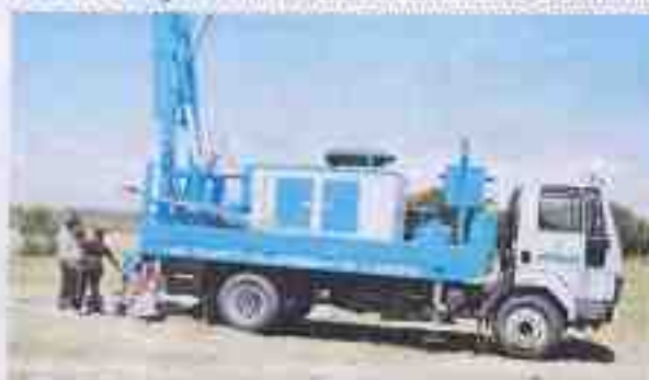
Borehole Drilling - CAIP Rumuruti Ward
